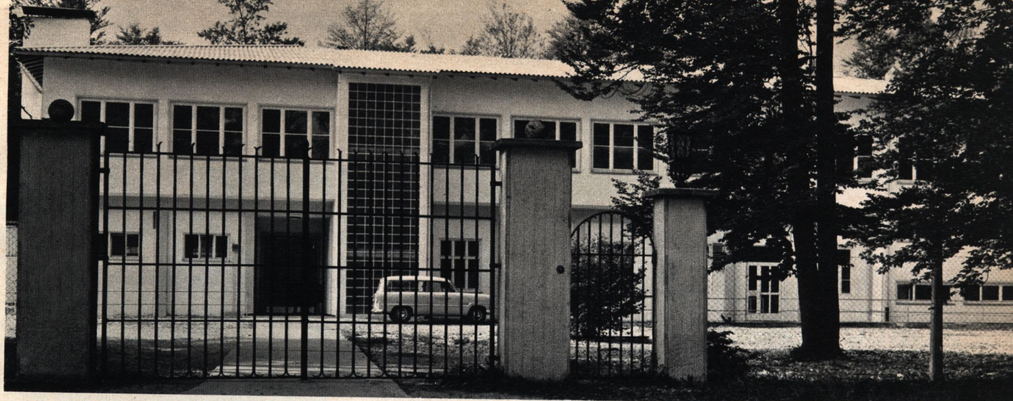
LINHOF tripod factory at Wolfratshausen/Gartenberg.
