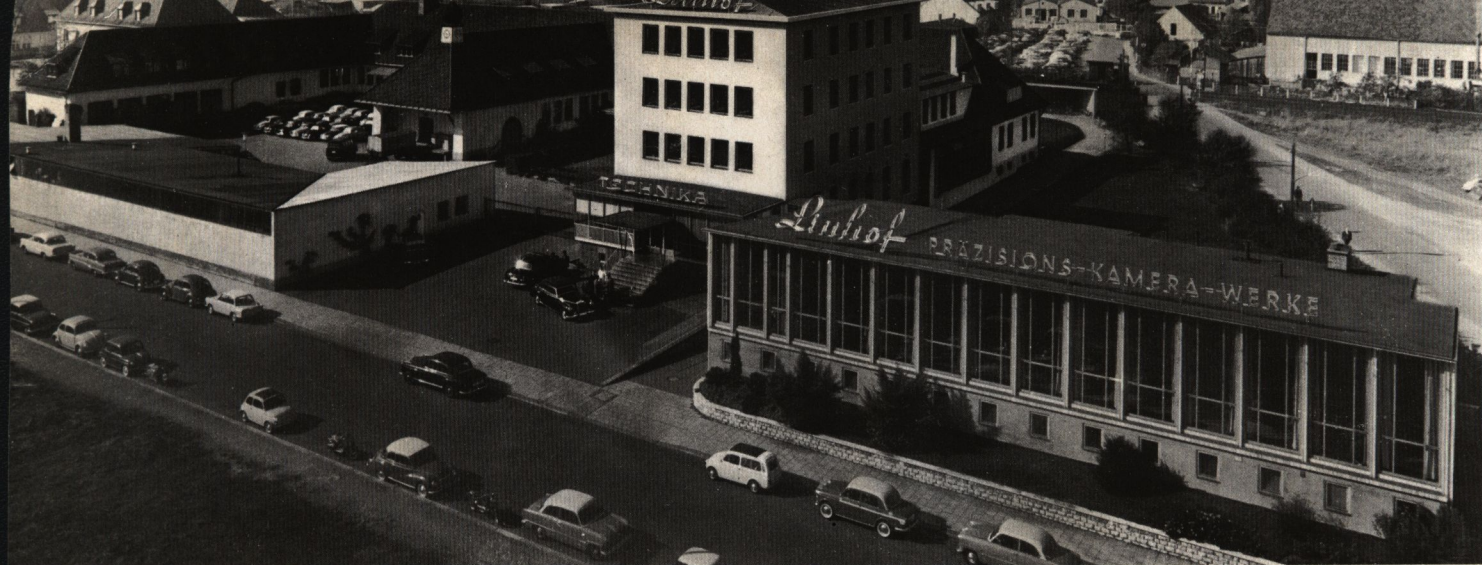
Main factory and administration offices of Linhof, Nikolaus Karpf KG, at München-Obersendling
