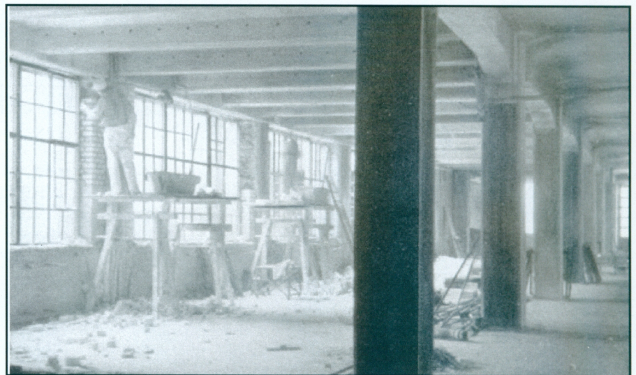
Two views of the work in progress to restore the workshops to the condition necessary to resume operations.
