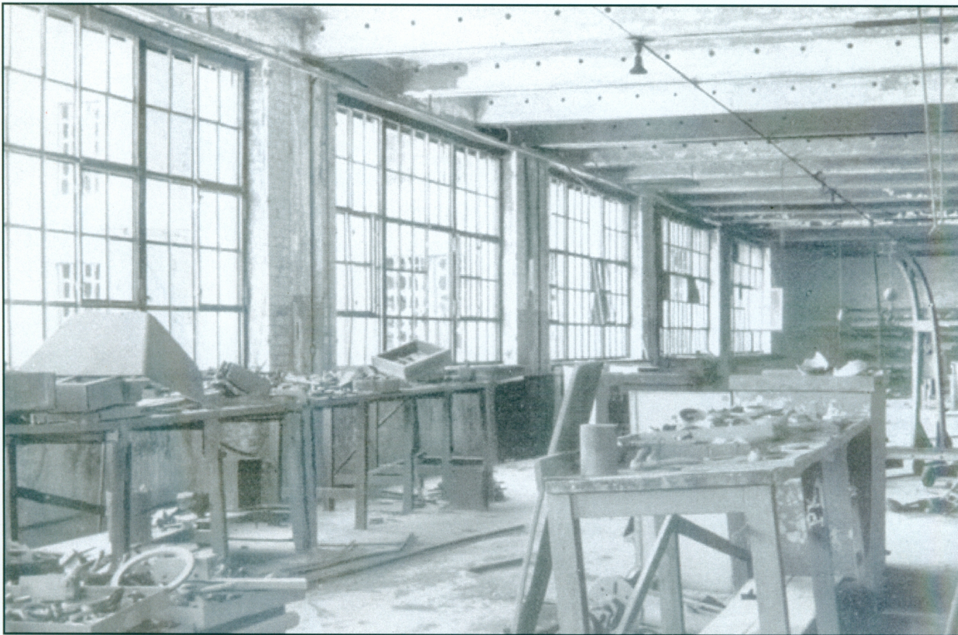
After the dismantling, only the old workbenches and these few useless scraps were left behind.
